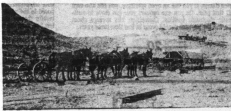
Team power Wagons haul pipe at a railroad construction site between Lubbock and Coleman in 1910. Teams are hauling the pipe on specially-built wagons by Studebaker.
