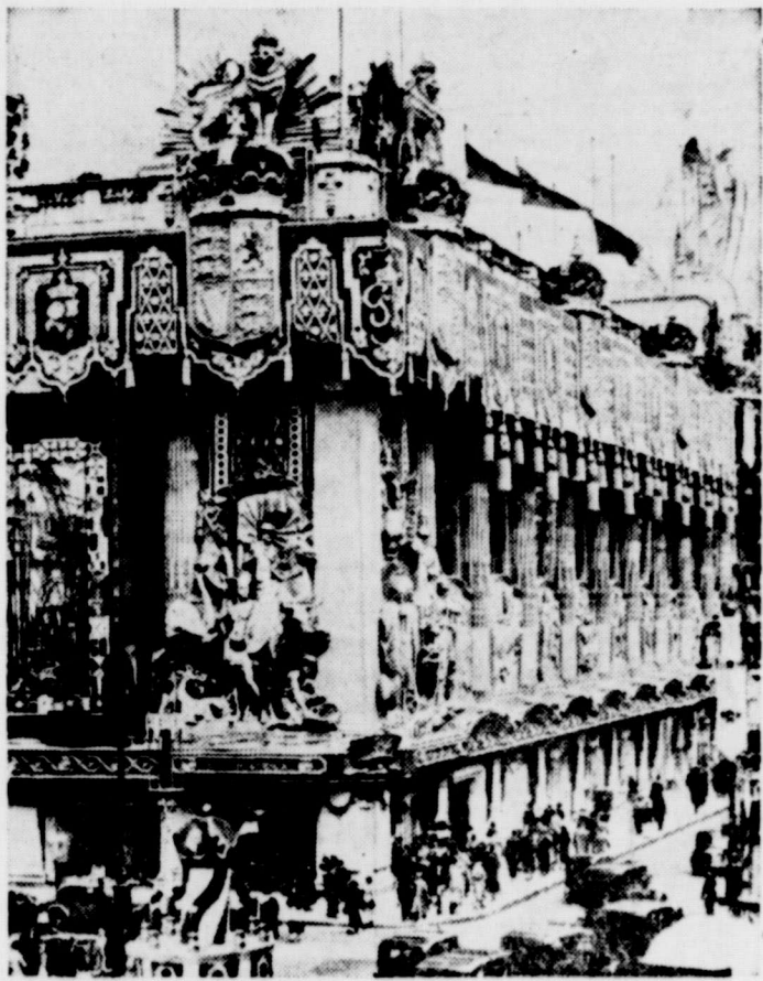
Can you guess what sort of building this bit of highly ornamented architecture is? Don't feel chagrined if you don't know right away that it is a department store. The special decorations to commemorate the coronation of King George VI coat Selfridge's in London $125,000 and nearby concerned the structure with a profusion of statuary and murals.
