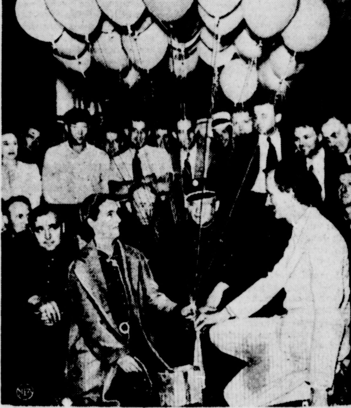
His new stratosphere craft looks like an inverted bunch of grapes. Dr. Jean Piccard explained to Mrs. Piccard and a ground crew as this picture was made at Rochester, Minn., where the stratosphere balloonist will take off on his next flight. Instead of one bag, the flight will be made with eighty four-foot balloons filled with hydrogen.
