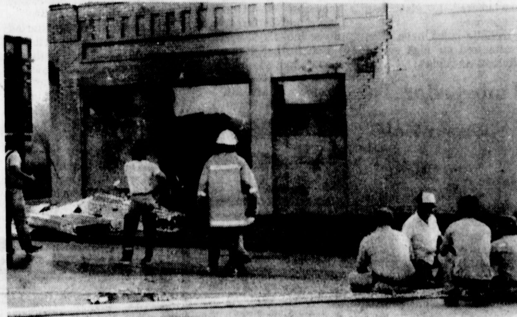
Cisco Volunteer Firemen Assessing Fire Damage
