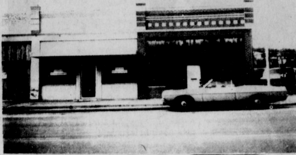
SHOWN IN THE ABOVE photo is the new City Hall and Police Station, located at 500 and 502 Conrad Hilton Avenue. There will be an Open House Friday, March 16, from 9 a.m. till 4 p.m. (Staff Photo)
