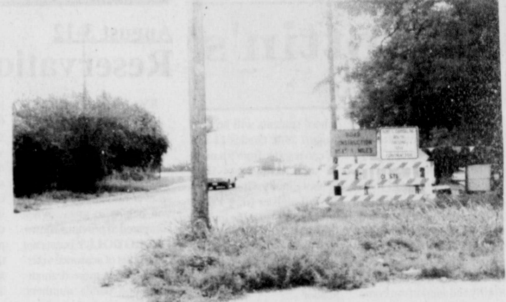
Signs near the Leon bridge on East Main in Eastland warn motorists of construction from the bridge eastward to the I-20 overpass. The heavily traveled route will be very dangerous while its being renovated, so motorists should slow down and be careful.
