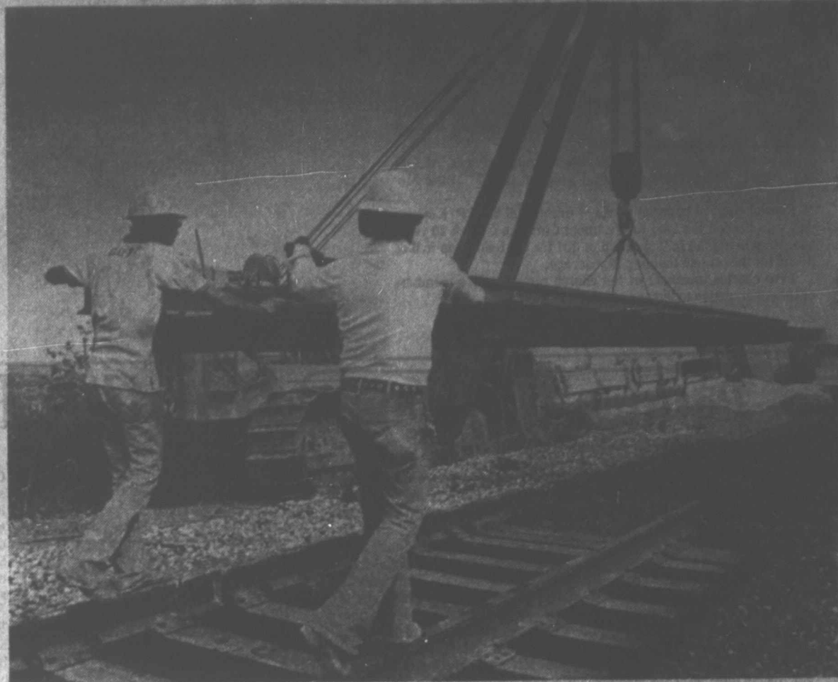
Moving the track into position
