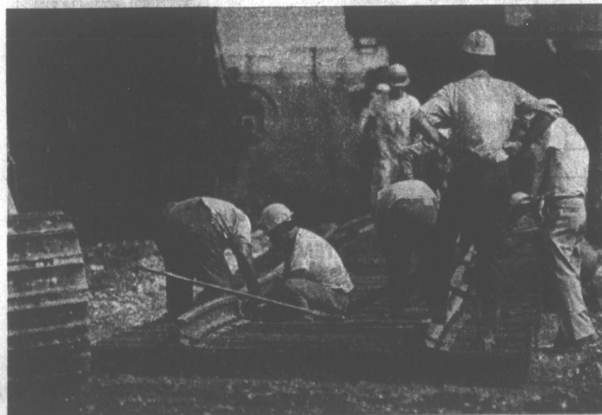
Placing the track into position
