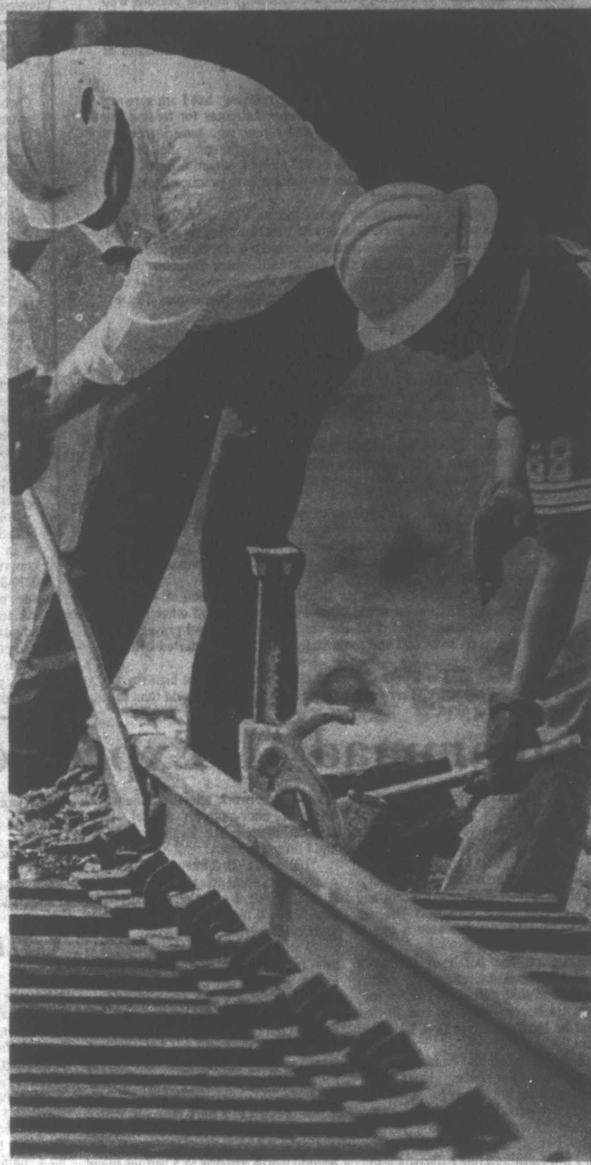
Aligning the track
