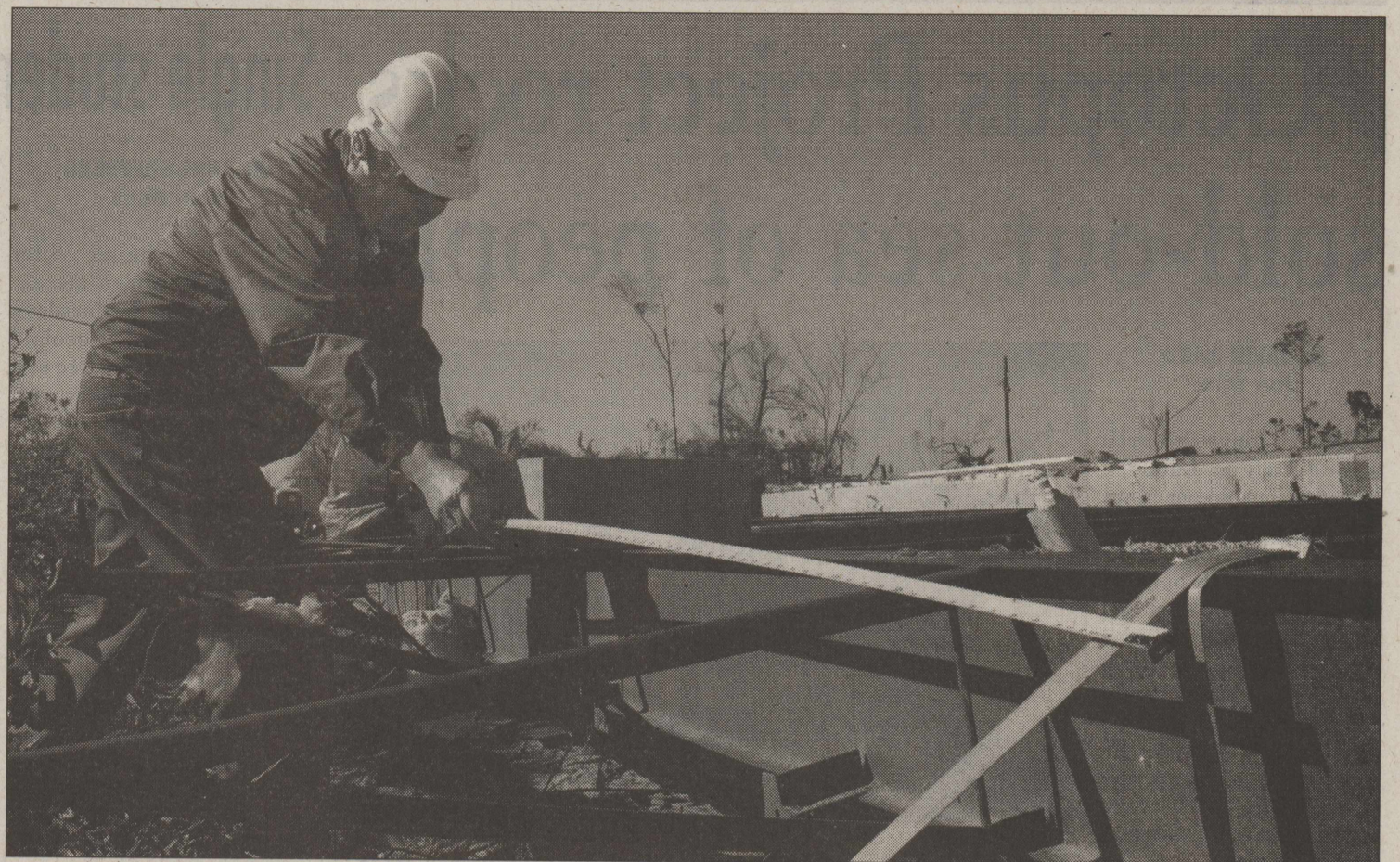
LARRY TANNER, MANAGER Debris Impact Facility/Research Associate from the Wind Science and Engineering Research Center at Texas Tech University, takes measurements of the tie down straps on the frame of double wide in the Lake Mack area that was destroyed by a tornado. Researchers from Tech visited areas of Central Florida that were damaged by the storm.
