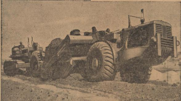
**CONTRACTORS' PET**—These two International earth-moving giants are favorites of contractors who want to move tons of earth in a hurry at low cost. This big 262 h.p. International Model 75 Payscraper, capable of hauling 22 cu. yds. of material at speeds to 24 m.p.h., is shown being push-loaded by another favorite of contractors, the International TD-24 diesel torque converter crawler tractor which develops 200 net engine h.p.
