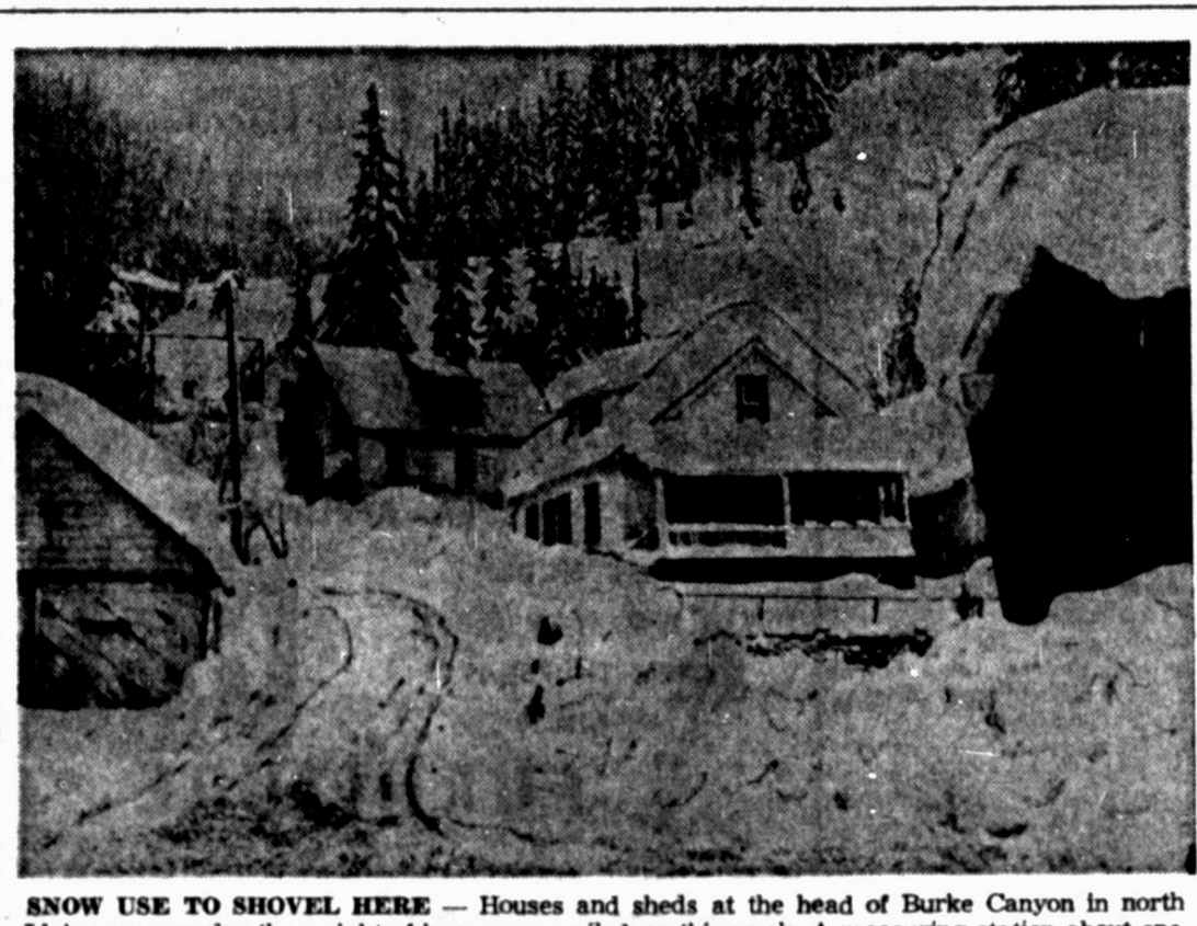
SNOW USE TO SHOVEL HERE — Houses and sheds at the head of Burke Canyon in north Idaho groan under the weight of heavy snow piled up this week. A measuring station about one mile up the canyon gauged 81 inches of snow Wednesday. Residents are watching for possible snow slides, recalling an avalanche that took two lives on Jan. 5, 1933. (AP Wirephoto)
