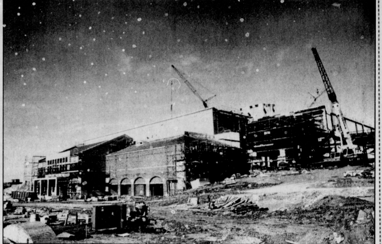
United Spirit Arena construction
