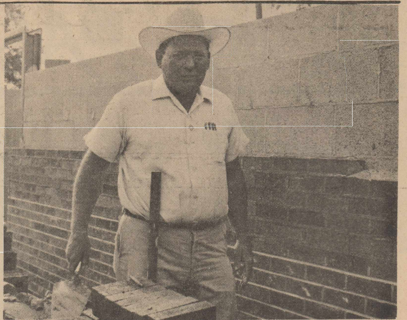
Eugene McCown was given a $25.00 saving bond at the Noon Day Lions Club Tuesday for a show of appreciation for the five or six days donation of time for building the concession stand at the Little League Park. The building is 10' X 20'. He is shown here working on a 'Raymond Buhman Construction Job' across the street from the Post Office. This is another example of Seminole "on the move" and growing. This new addition will certainly add to the downtown area.
