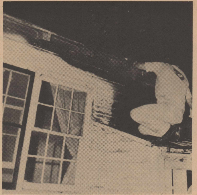
WAYLAND MCCULLOUGH STANDS ON AN OUTSIDE LEAN-TO BUILT FOR A HOT WATER HEATER AND CHECKS THE FIRE AT 301 S.W. 4TH ST. AT 10:05 P.M. MONDAY. THE FIRE HAD STARTED FROM THE HOT WATER HEATER IN THE SMALL ENCLOSURE. DAMAGE WAS NOT TOO EXTENSIVE. THE INSIDE STRUCTURE RECEIVED NO DAMAGE. THE HOUSE WAS OCCUPIED BY THE JOE CALDWELL FAMILY.
