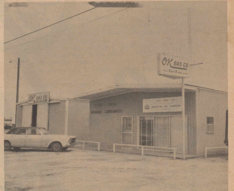
O K Gas Company, South Main Street.
