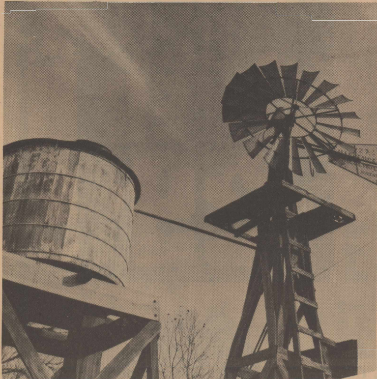
THIS IS WEST TEXAS - - - A windmill still in use on the D. P. Williams farm, just north of Seagraves - a No. 27 Hallowell, built in Batavia, Illinois and sold by Higginbotham-Bartlett Company.
