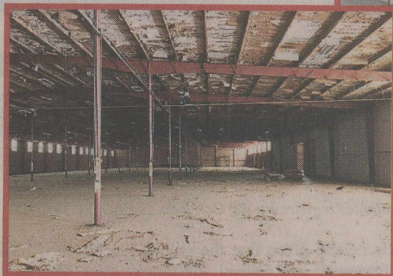
The "before" picture of the Tye Manufacturing Plant building.
