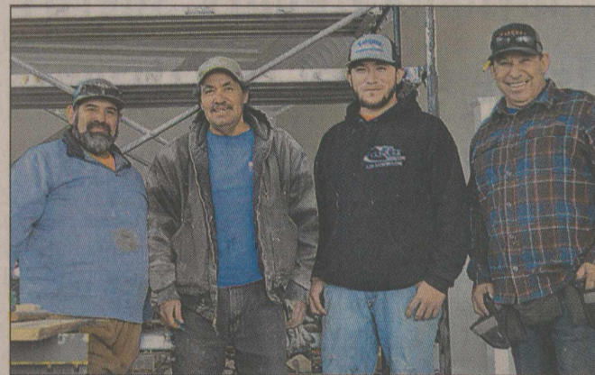
BARROW BUILDING-Ricky Vasquez of Vasquez Roofing and Remodeling (Lockney) and his crew have transformed the interior of the Barrow Building that sits on the north-west corner of Floydada's downtown square. Notice the ceiling detail-it has been restored and painted. The crew was gathered allowing me to snap a photo of them during a recent work-day. Pictured above (L to R): Robert Gonzalez, Nacho Mondragon, Ricky Vasquez Jr., and Ricky Vasquez (owner). Call Ricky at 806-292-6742 for your next roofing and remodeling job.
