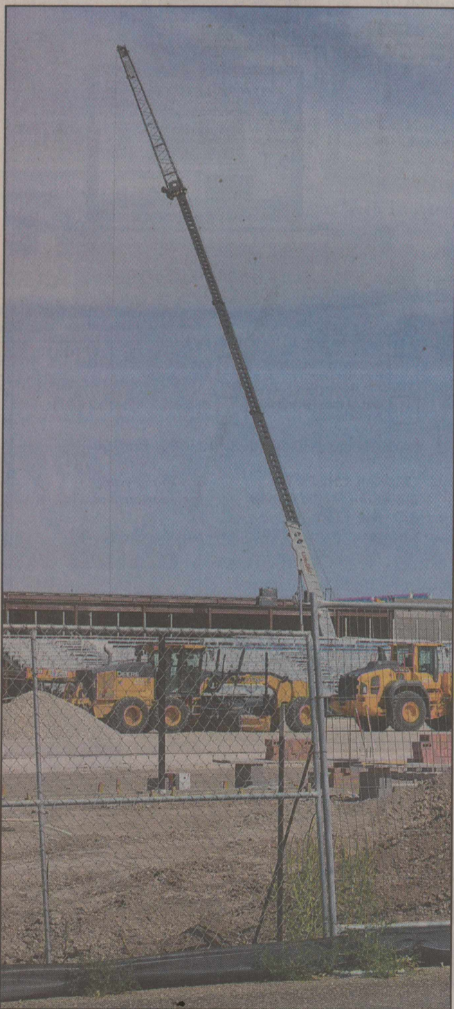
FHS Dirt Work on Field
