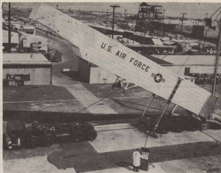
TRAILER FOR MINUTEMAN —The Minuteman ICBM can now be carried to its underground launch site by this 63-foot-long truck container. When the container is upright, a hydraulically powered hoist, capable of handling 50 tons, gently lowers the missile into its underground bed.
