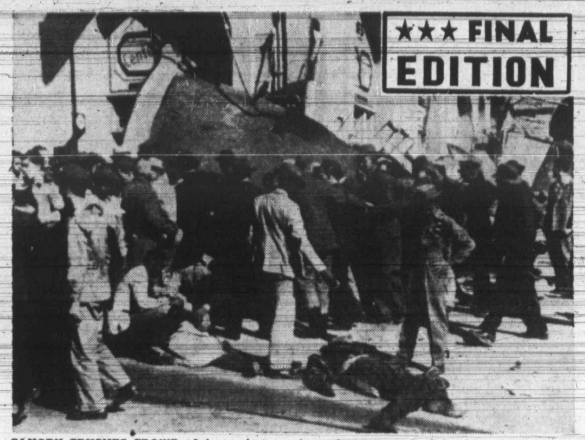
CANOPY CRUSHES CROWD—A large plaster and wooden canopy, loaded with spectators at an Armistice day parade in Houston, collapsed and crashed into a crowd standing beneath it. Two men were killed and 50 other persons injured. 14 seriously. Marching soldiers immediately broke ranks and aided police in holding back the huge crowd and removing victims. Note body of one of the persons killed lying on the curb while first aid is administered to another at left.
