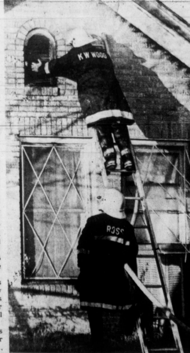
FIREFIGHTERS AT WORK—Snyder Firefighters battle a blaze that heavily damaged a dwelling at 2805 Ave. M late Tuesday. The inside of the house and its contents were a shambles before the blaze was extinguished. (SDN Staff Photo)
