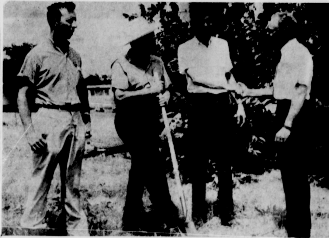
CONSTRUCTION TO BEGIN — Hal Hayes, local manager of Community Public Service, mans the shovel as Skeet Fambro, area CPS manager, far right, and Billy Averett shake hands as negotiations were completed Friday
