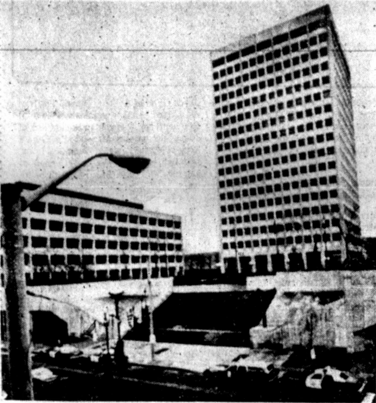
CONTAMINATED BUILDING — The state office building, the tallest building in downtown Binghamton, N.Y., stands empty more than a month after an explosion spewed some of the deadliest chemicals in the world through its 18 stories. Officials are unsure how to clean up the mess. (AP Laserphoto)
