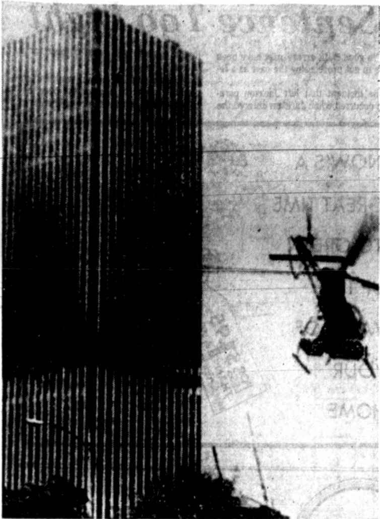
INFERNO KILLS 11 — Fire erupted Saturday from this 36-story office building in Santiago, Chile killing 11 and trapping dozens more on the upper floors. Police helicopters evacuated those trapped from the roof of the building. (AP Laserphoto)
