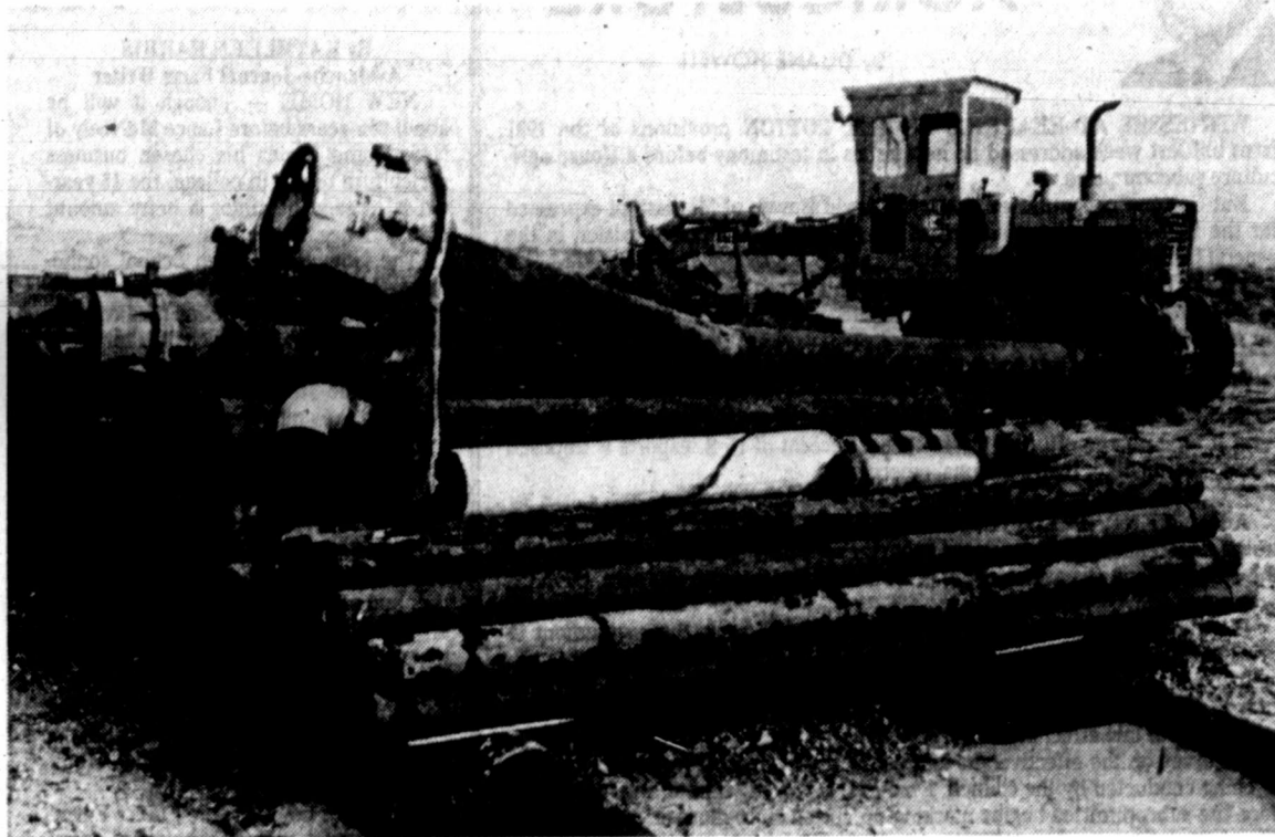
Water Pipe at Lubbock Pumping Station Near Muleshoe
