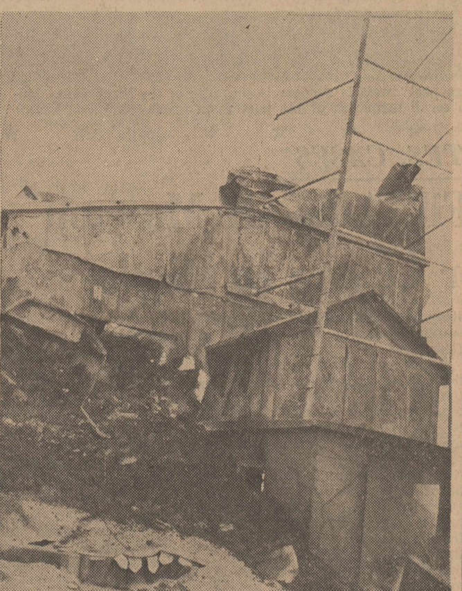
spilled debris and smoldering grain on the east side of the large complex. Damage was estimated at $70,000. Fire still smolders on the west side of the crumpled structure in the right photo, hours after the blaze broke out. (Staff Photos by Tanner Laine)
