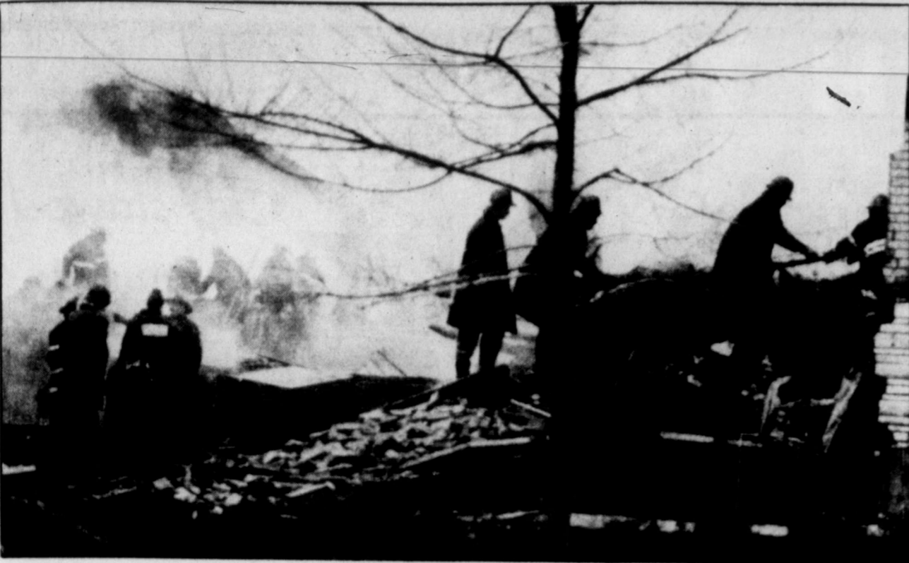
Montreal firefighters begin sifting through the debris following an explosion Tuesday.
