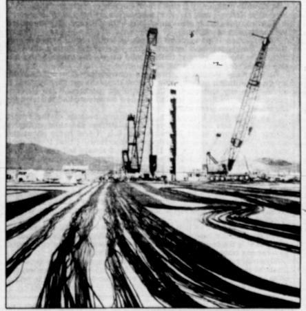
Dozens of electronic cables that will transmit data from a nuclear test at the Nevada Test Site snake toward a drill site.
