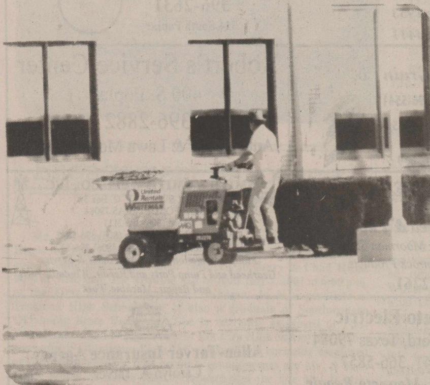
Shown above and at left: Workers in the process of hauling dirt in to the school to fill up the auditorium before pouring cement.
