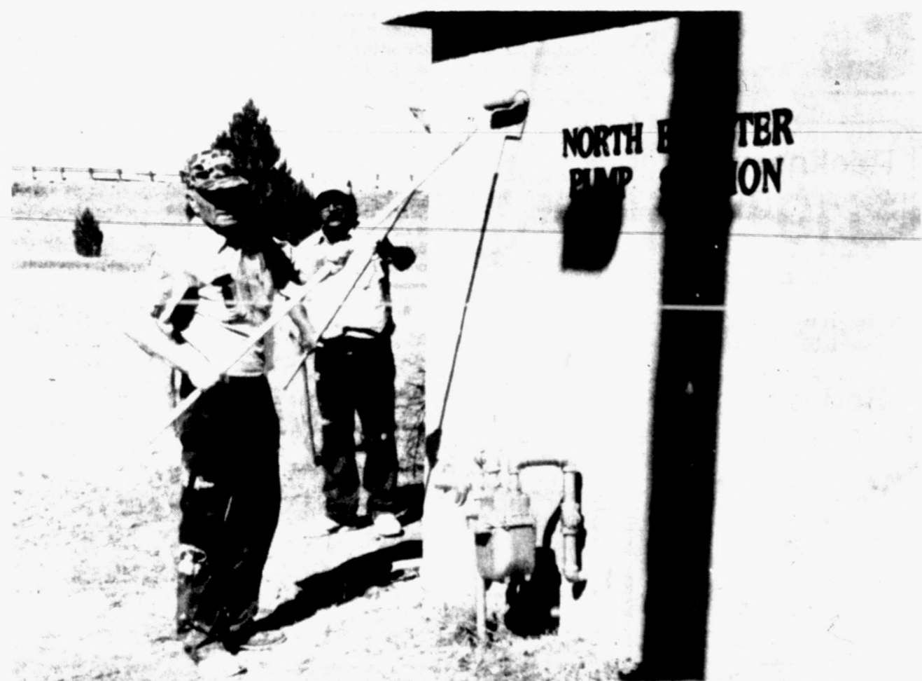
FINISHING TOUCHES — Kenneth Rinehart, left, and Raymond Valadez complete the painting of the outside of the North Booster Pump Station. Painting and repair work is also in progress at the W.S. Bigham Water Treatment Plant. (SDN Staff Photo)
