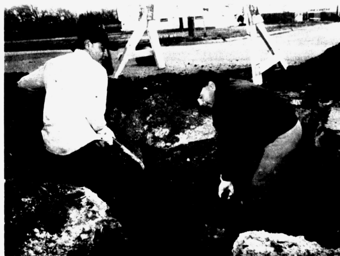
PROJECT BEGINS — City employees Roger Smith and Ricky Sosa dig around a portion of the Ave. T water line as rehabilitation work begins. Line rehabilitation includes flushing the line and then adding a cement lining. City officials said they would begin laying temporary water lines to service affected customers today. (SDN Staff Photo)
