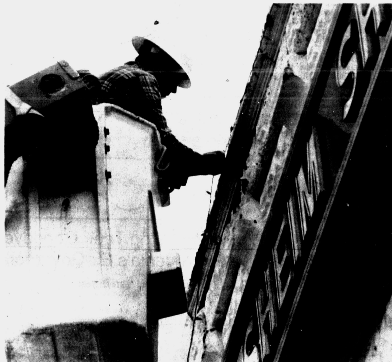
STRINGING LIGHTS —Thomas Whitt of Midwest Electric strings lights along the tops of buildings around the square this morning. Multi-colored lights will outline the buildings as white lights silhouette the courthouse for the chamber's "Light Up Snyder" project. (SDN Staff Photo)
