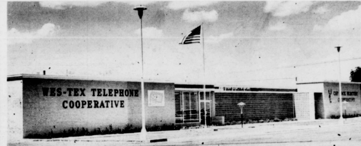
CAP ROCK TO HOLD OPEN HOUSE — Two of Martin County's largest businesses will give area residents an opportunity to visit and see the beautiful new building at an Open House here Sunday afternoon from 1:30 p.m.
