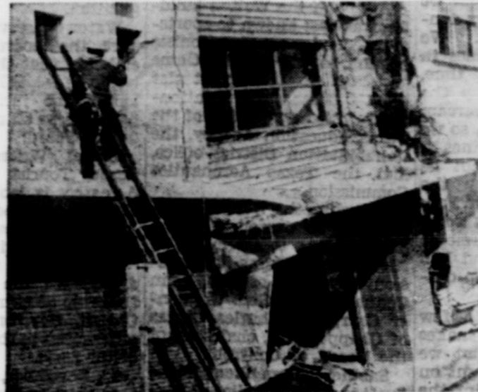
RESCUE CHIEF for Anchorage Civil Defense, Bill Hendricks, smashes through a window prior to entry into an apartment building to search for victims of the earthquake which devastated Alaska on March 27. A soldier on guard duty reported hearing cries for help earlier, but no victim was found. Hendricks personally removed two dead victims from the ruins of buildings.
