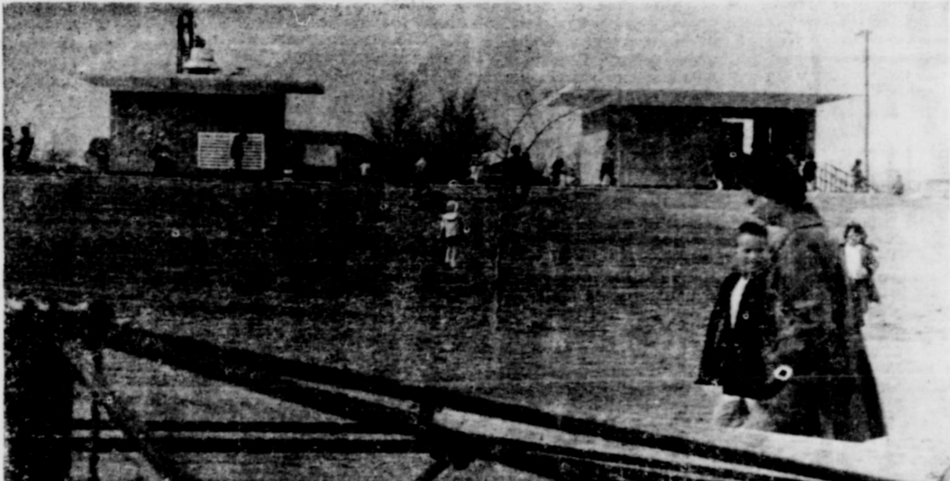
ENTRANCE TO THE CAVERNS—Stanton's new underground school, referred to by older students as the "Cavern", was put into operation Friday when first and second grade classes moved in. The building on the right is an entrance hall. Structure at left is a maintenance room. Eight classrooms lie under the two structures.
