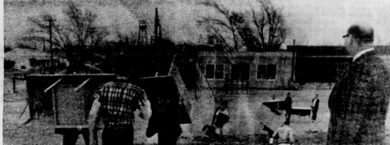
OUT WITH THE OLD—Stanton students played the part of movers Friday morning and shuffled furniture from the old school building to the new underground structure. The moving process continued until noon Friday when first and second graders settled down in their new rooms. Beryl Clinton right, superintendent of schools, directed the moving process.
