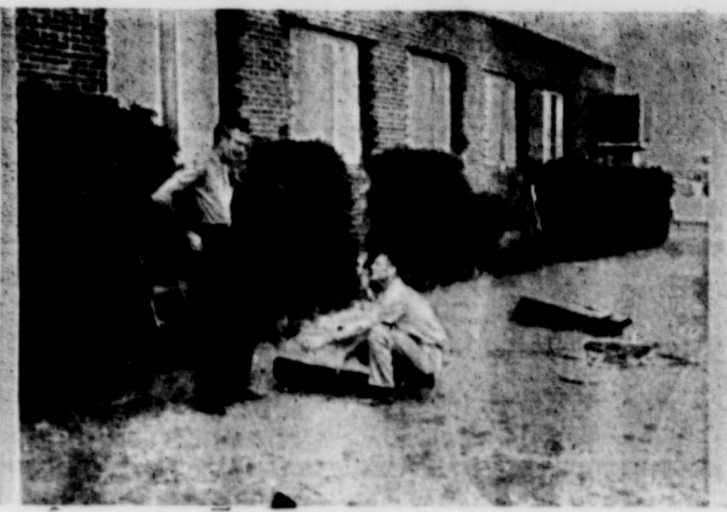
MINISTER AND CONTRACTOR —Doyle Corder, minister of the Church of Christ and Guy Fink, contractor, are shown on the lawn of the church. New windows are being installed and other church improvements are planned.
