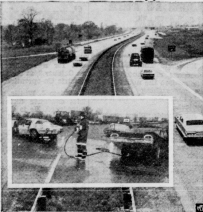
Twenty grinding head-on collision fatalities occurred on a seven-mile section of the eastern end of Mich- igan's Interstate 94 in the neighborhood of Ypsilanti when speeding vehicles crossed over the narrow median separating opposing traffic lanes. The long reign of terror on "Death Row" stopped abruptly when the Michigan Highway Department installed a double safety barrier of resilient steel in the narrow median. Inset shows a typical cross-over accident which brought tragedy before guard rail. It is unlikely to pay a return call on the now protected median (above).
