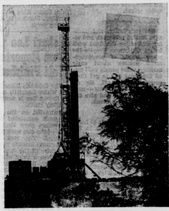
DRILLING THE DEEPEST Humble Oil & Refining Company's Rig 32 is shown here in the Gomez field of West Texas drilling the world's deepest producing well. The new ultradeep producer—the Henry Willbanks No. 11—was completed in the Ellenberger formation at 21,883 to 22,610 feet. The well, located in Pecos County about 10 miles northwest of Fort Stockton, flowed gas at a calculated open flow rate of 14 million cubic feet a day.
