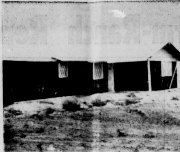
THE LEDBETTER HOME. Set off from Hwy. 80 a short distance is the Alton L. Ledbetter residence under construction in the western area of Stanton.
