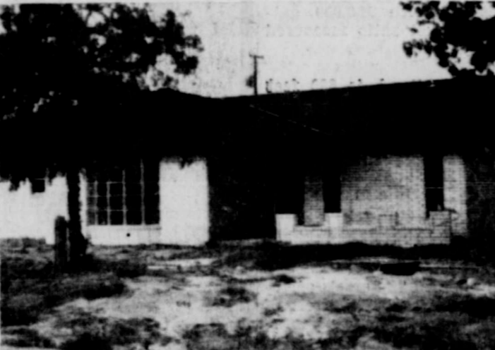
JIMMY JONES HOME. The new residence for Jimmy Jones is shown here with an imaginative design and convenient facilities.
