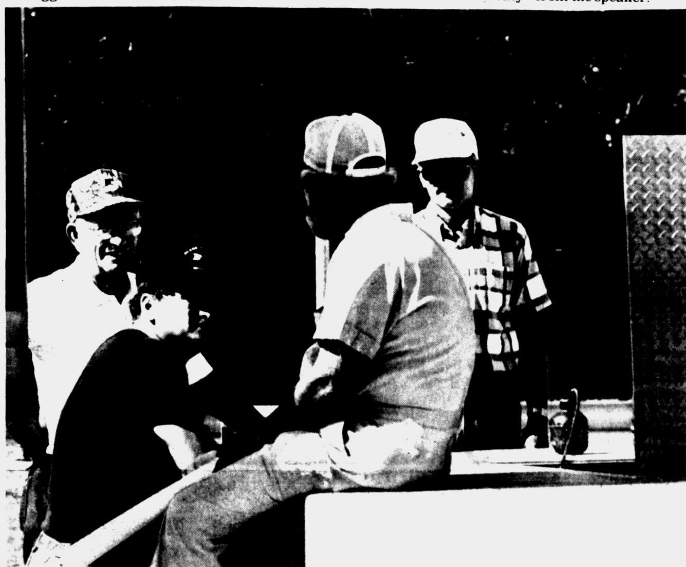
LIFT STATION — City officials and Panhandle Construction Co. owner Dave Hampton of Lubbock, left, Wednesday filled the new sewer line to the Price Daniel Unit with water to test the lift station on 37th St., pushing the water to the top of the hill to the west, where gravity carried it on to the
