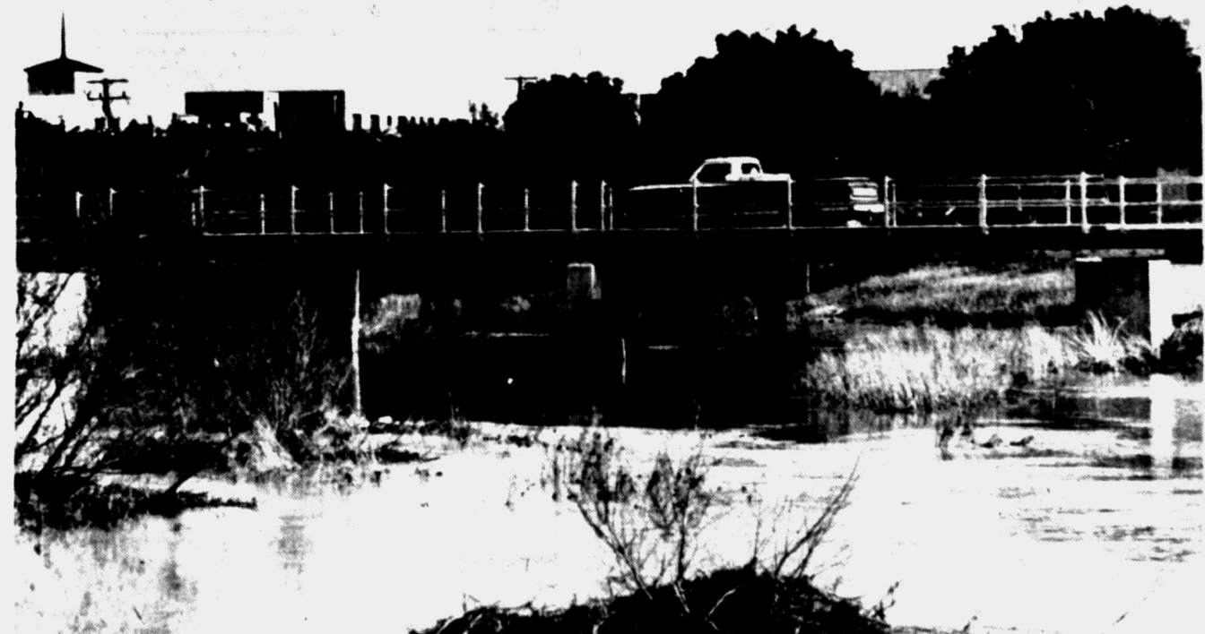
CREEK LIKE A RIVER — Deep Creek looked more like the Colorado River Friday morning following reports of up to 5 inches of rain Thursday night on the Fluvanna area watershed. The storm
