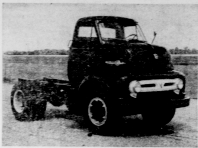
Ford engineers claim these newly-designed C-150 Series cab-forward trucks set a pattern for the industry with their wider, 3-man cabs with full-width seats. They have greater maneuverability and shorter turning radius; new, curved, one-piece windshield with 55 percent more visibility and 4-foot wide rear window. Synchro-silent transmissions do away with double clutching. This new cab-forward design makes possible almost all engine service operations from the front of the truck.
