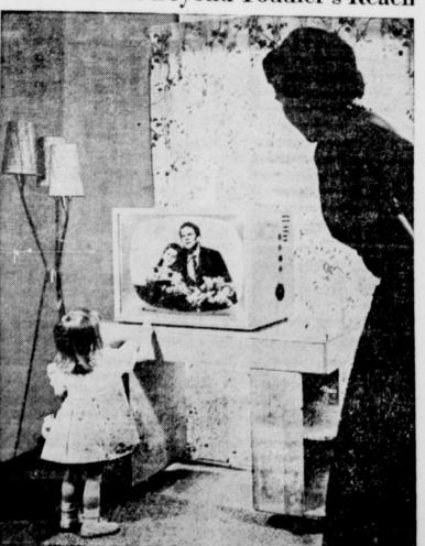
Primary controls of Crosley's compact new 21-inch Super V television receiver are mounted conveniently together on the right side of the set in easy reach of the operator, yet well beyond the range of toddlers. Using a revolutionary short aluminized picture tube the new 21-inch set gives up to 30 per cent more viewing area in 23 per cent less space than ordinary 21-inch models. Set actually takes no more cabinet space than ordinary 17-inch models.
