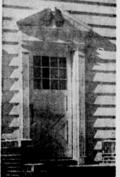
This panel door is one of many authentic designs dating from the 18th Century and earlier. The stately frame with its "broken pediment" on top and square columns is typical of fine old homes in New England, Virginia, and the other colonies. Both door and frame today are stock ponderosa pine millwork items, eliminating the need for custom millwork.
