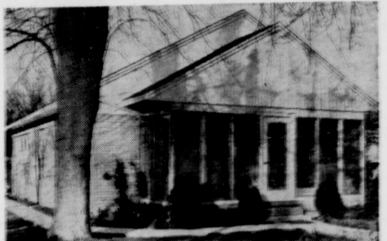
Size and location are the only two features the attractive remodeled house, above, has in common with its predecessor, right. A clean new roof line was the key to the improved appearance. The porch became a sun-room and its roof was raised to be consistent with the main roof.
