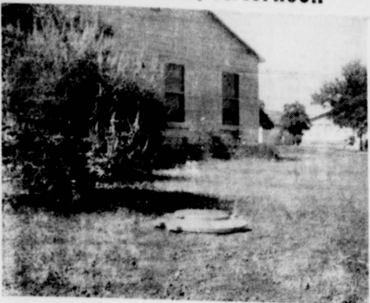
This view shows an underground, sanitary garbage container installed at a home here in Burkburnett. Note how the container blends in with the grass, shrubs and other surroundings. They can be installed either in the front, back or beside the home. The outside container is made of fiberglass. The removable, inside container, is polyethylene.
