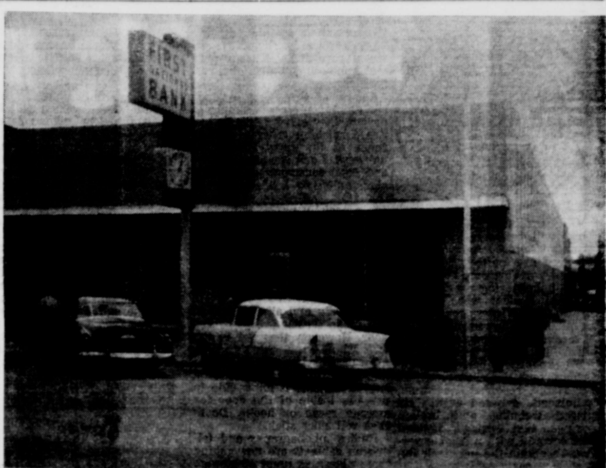
Front of the First National Bank. The new addition is walled with Roman brick and cast stone to harmonize with the existing bldg.
