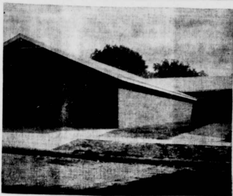
The new Educational Building just completed for the Church of Christ. The new addition has 11 classrooms, (20 persons per classroom capacity), and a library. This gives a total of 26 classrooms for both buildings. The church has 44 teachers. Each classroom is complete with individual student desk art chairs.
