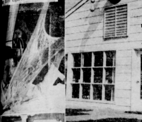
LOOK OUT below! You can never tell when those hanging drops, rigged by a resourceful Central States plumber, will fall.
