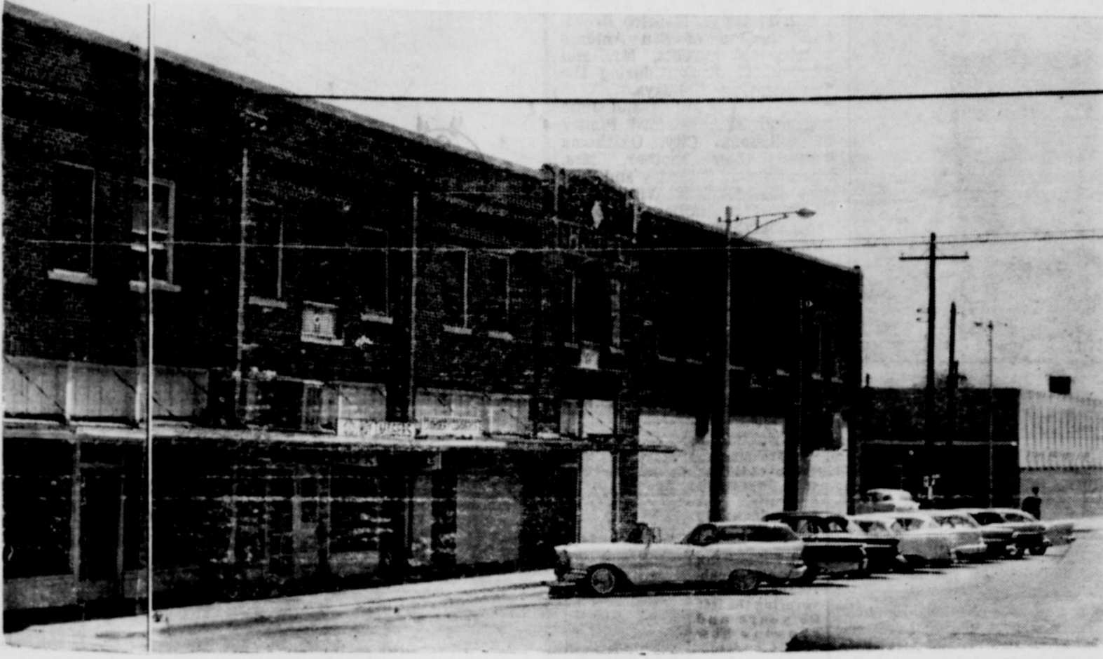
Above is shown the old hotel or Collier Building as it looked before work was begun for new offices, dining room and kitchen, and display space for Texas Electric Service.
