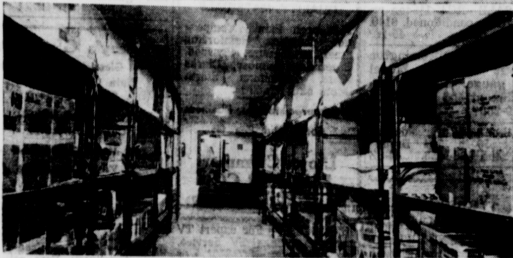
EMPLOYEE SHELTER built by the Marotta Valve Corp. of Boonton, N. J., under the home (top) of its president is often cited by civil defense authorities as an example of what a smaller firm can do to protect itself and its workers in the nuclear age. The main room (below) of the self-contained shelter is stocked with a 30-day supply of all necessities for 100 persons. All of the company's nearly 200 employees could be sheltered in the private structure within six minutes after warning of a possible attack was received in the nearby plant.
